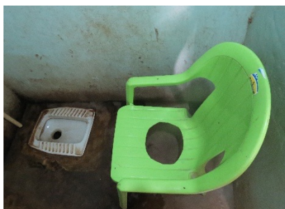
Figure 3. Examples of latrine seats, water point ramps, and improvised brick handrails from disability project in Mali (see Appendix E1 )
