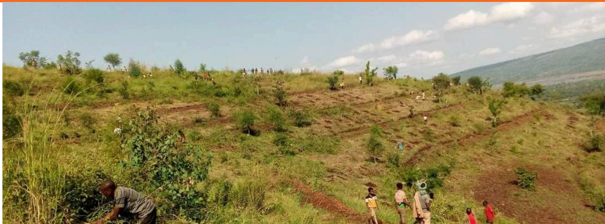
Habro woreda, Bareda kebele, Gara Adayo watershed (trenches)
