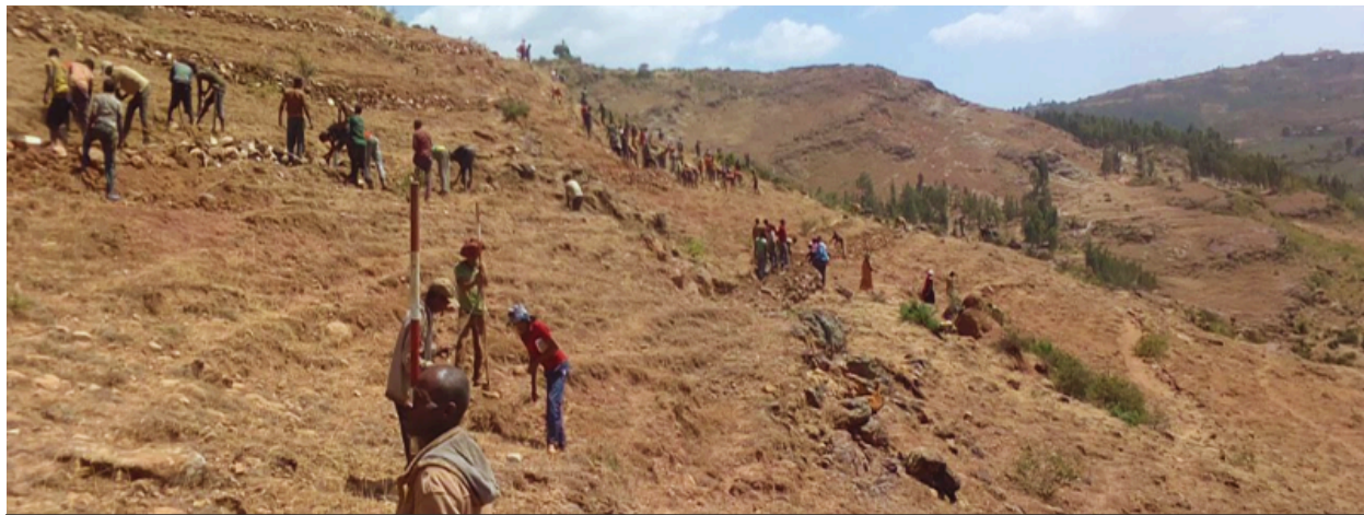
Habro woreda, Oda Anani kebele, Setegn watershed Ayo area closure (protected from human and livestock disturbances and hillside terraces)
