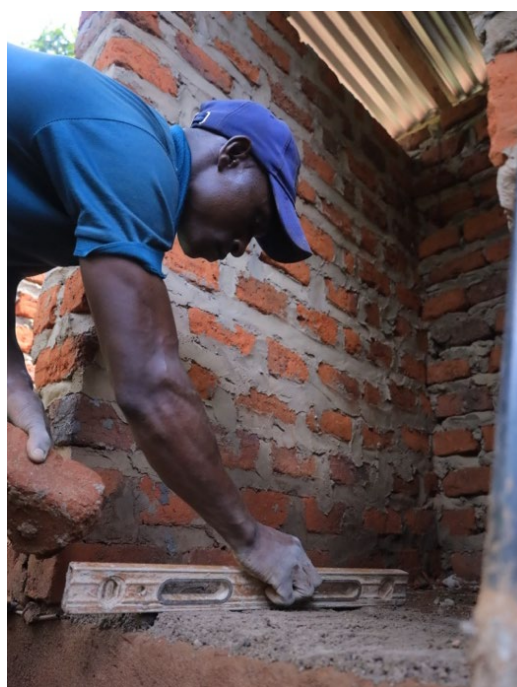
A mason constructing a washable floor in a pit latrine
