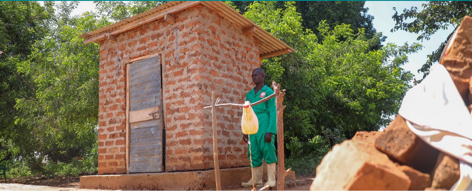
A mason next to a newly constructed pit latrine
