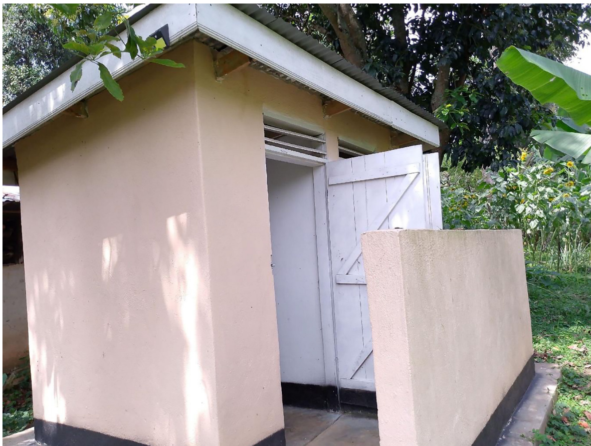
Figure 2.3. An improved sanitation facility constructed in Kyawakada Village, Kahangi Parish, Hakibaale Sub County-Kabarole District.
