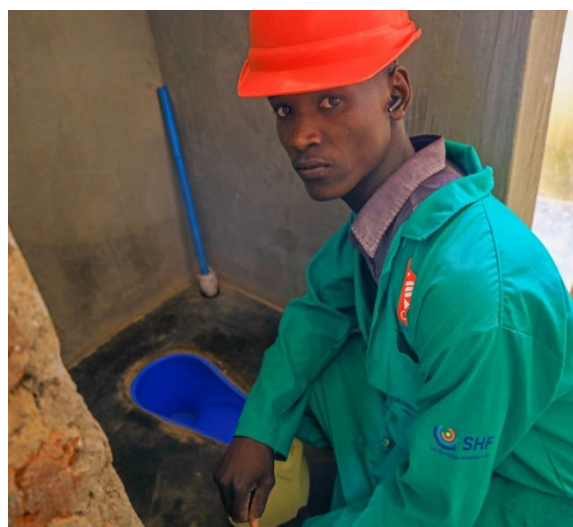
A mason next to an upgraded latrine
