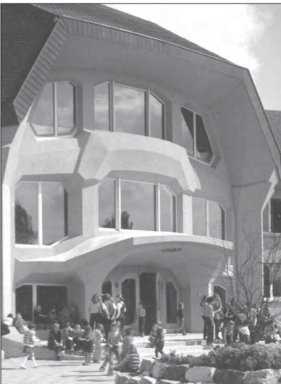
Figure 36. Rudolf Steiner School, Ittigen, front entrance.
