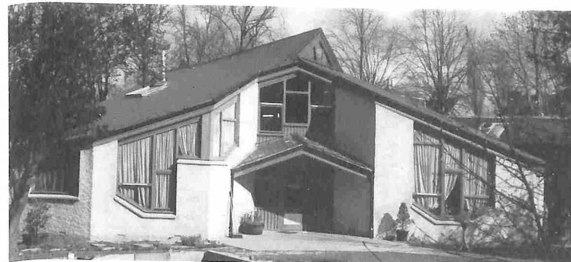
The new kindergarten of 'The Rudolf Steiner School of Edinburgh', Scotland. Architect: Wilfrid Bohm.
