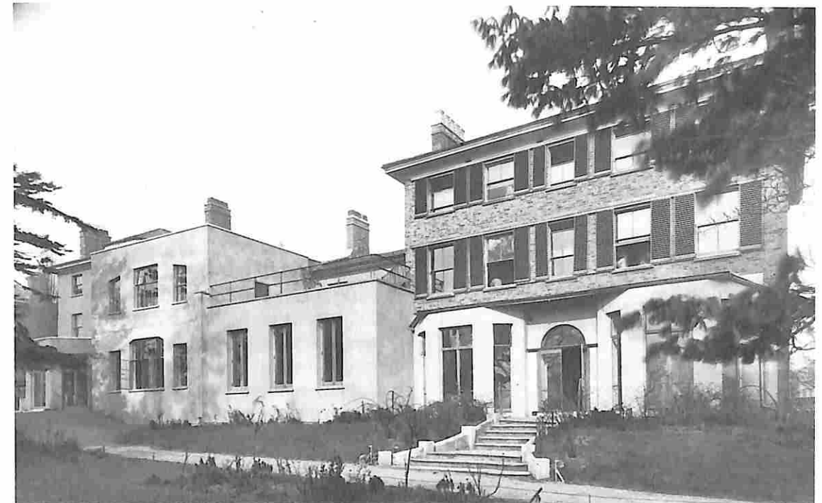
The 'New School': rear façade of the premises in Streatham, London during the early years of Waldorf education in the English-speaking world.
