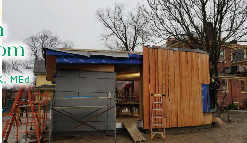
North wall in progress . . .
