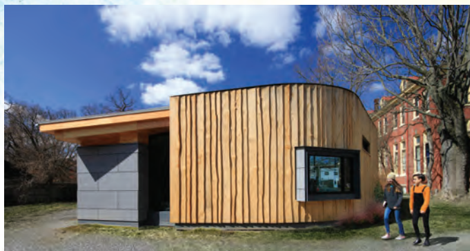
North wall completed with main school building in background to right
