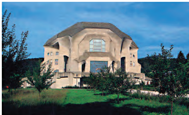
The second Goetheanum, Dornach, Switzerland, designed by Rudolf Steiner, is an example of his organic architectural style.
