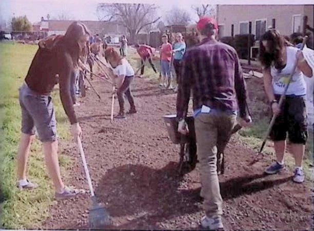
Community members and visiting volunteers work together to make a walking path usable and safe.
