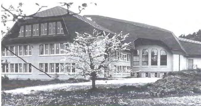
Rudolf Steiner School, Ittigen (Bern), Switzerland. Side view showing design kinship to nearby traditional Swiss farmhouse.
