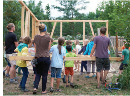
Students and parents help in the construction of a new Waldorf school in Dresden, Germany.
