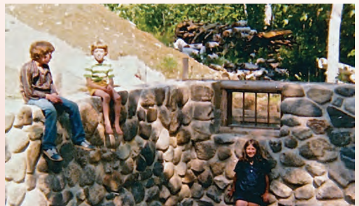
Rachel with brothers in the DIY stone foundation of their (in-process) family home
