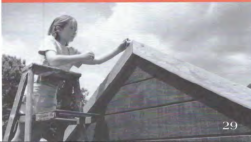
A student applies the finishing touches to the roof of a structure built by her class.
