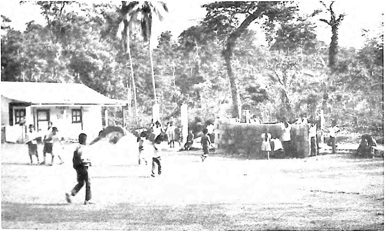
The school construction project, organized by the author, on a coffee plantation in Flores, Guatemala
