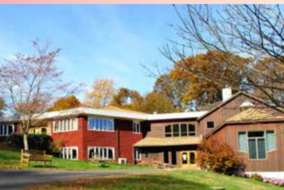
Classroom building, Camphill Special School, Glenmoore, Pennsylvania, constructed in 1975
