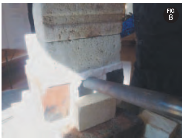
Figure 8: The building up the chimney at the front of the kiln.
