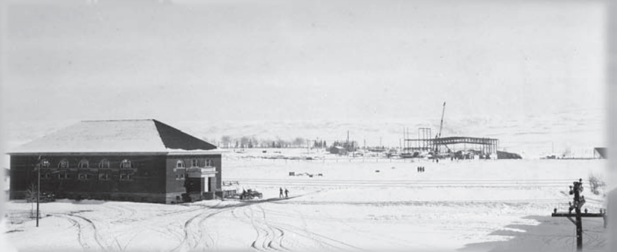
The Little Red Gym with Half Acre Gym under construction in the background, circa 1924.
