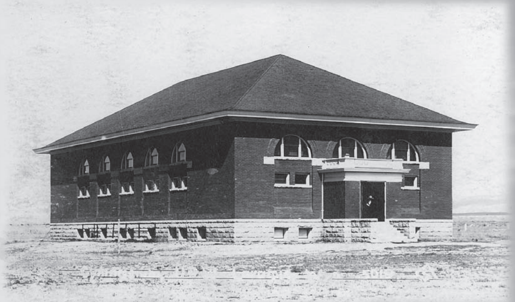
The exterior of the Little Red Gym.
