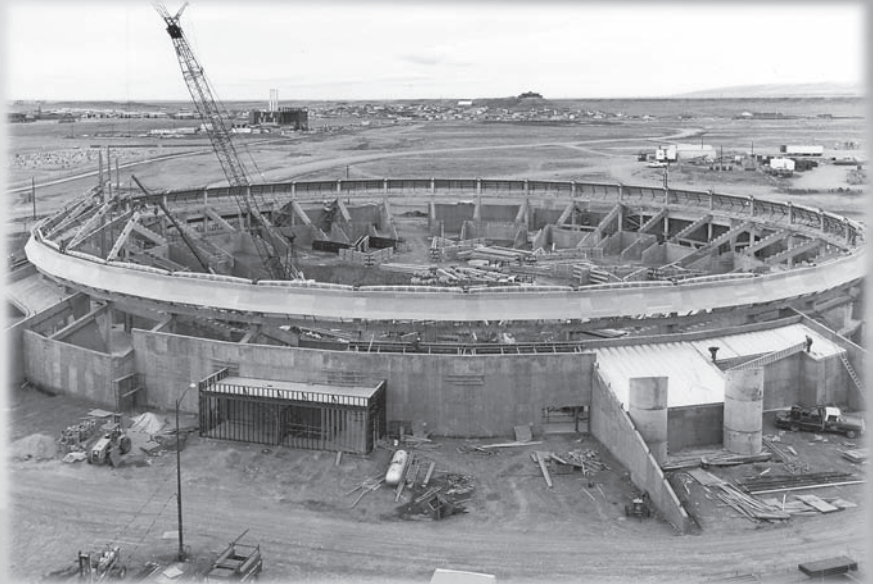
The Arena-Auditorium under construction, 1981.
