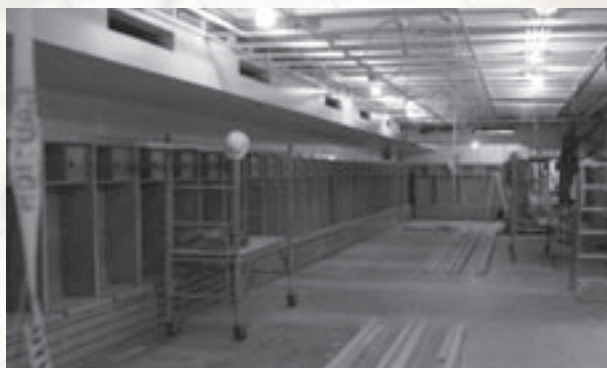
The new wood lockers being placed in the football locker room. When completed, all sports at Washburn will have updated locker facilities.
