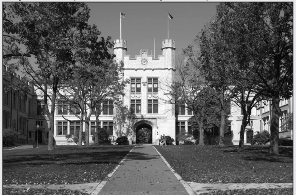
The interior of Wooster's primary academic building, Kauke Hall, was renovated during 2005-06 at a cost of $18 million.
