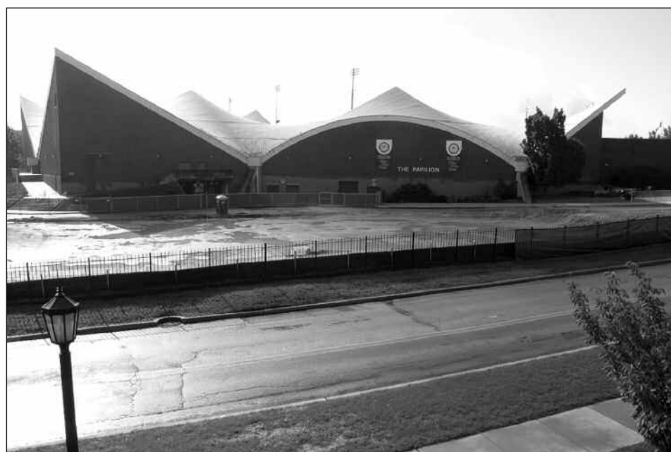
Construction began in July on the IARC, located directly in front of the Pavilion on Ithan Avenue.
