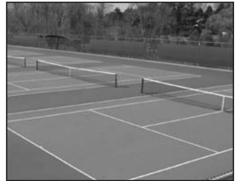
West Campus Tennis Courts
