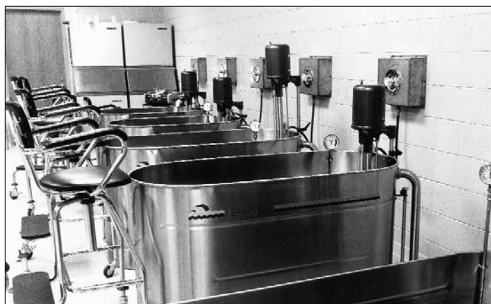
Tim Kerin Training Facility
