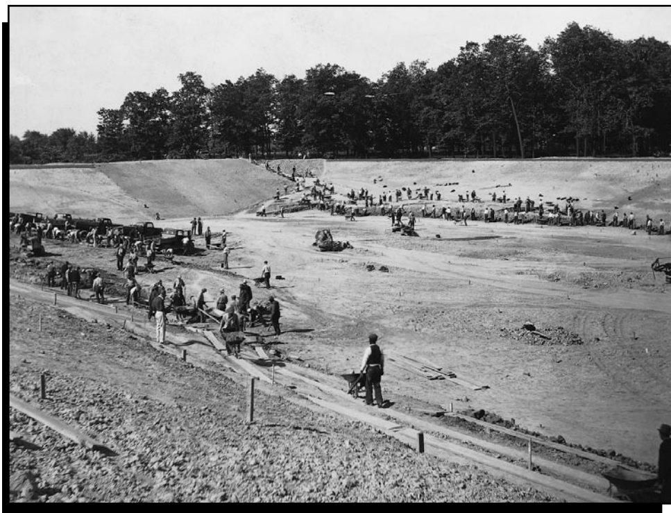
Construction on the Glass Bowl began as a WPA project in 1936.
