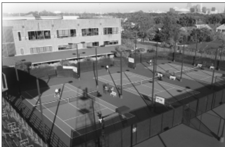
Home of the highly-successful Tulane tennis teams, the Goldring Tennis Center will be upgraded to add locker rooms and improved spectator views.
