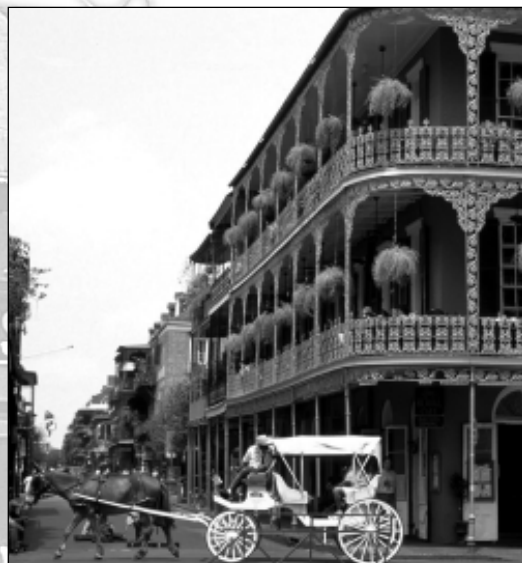
Nearly decimated by a fire in 1788, New Orleans' rich history is exemplified in the wide variety of architectural styles.
