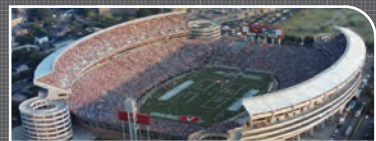
CAPACITY: 83,818 EAST SIDE UPPER DECK ADDED WITH TWO LEVELS OF SKY BOXES
