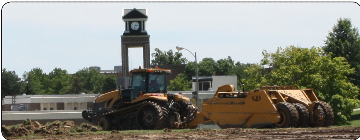
Heavy dirt work takes place on the construction site. The indoor facility will sit on the site directly in front of Spratt Stadium which was formerly the home of the MWSU Softball Complex. The main portion of the facility will sit on the area formerly occupied by Field Two, while a new 300-space parking lot will occupy the space where the main game field used to be.
