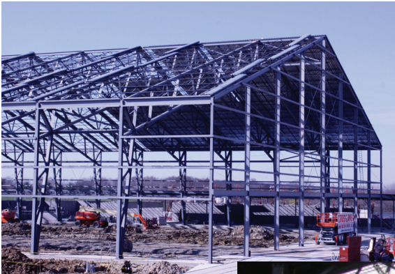
Above and Right: These images show the structure as it was going up, before the outside shell was put on. The pictures show the 17 columns that support the side of the structure, as well as the peak of the 73 foot ceiling in the center of the building.
