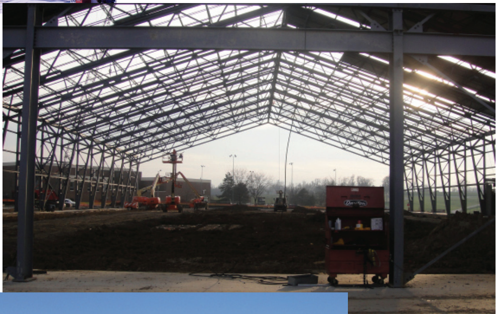
Above and Right: These images show the structure as it was going up, before the outside shell was put on. The pictures show the 17 columns that support the side of the structure, as well as the peak of the 73 foot ceiling in the center of the building.
