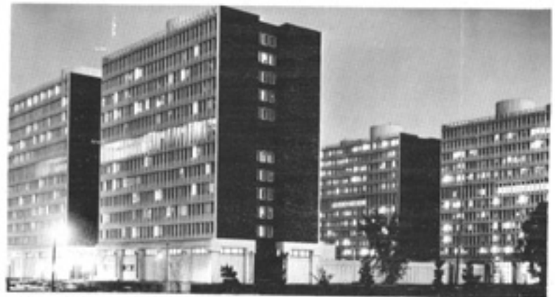
FOUR OF 18 new residence halls that have been built in the last decade.
