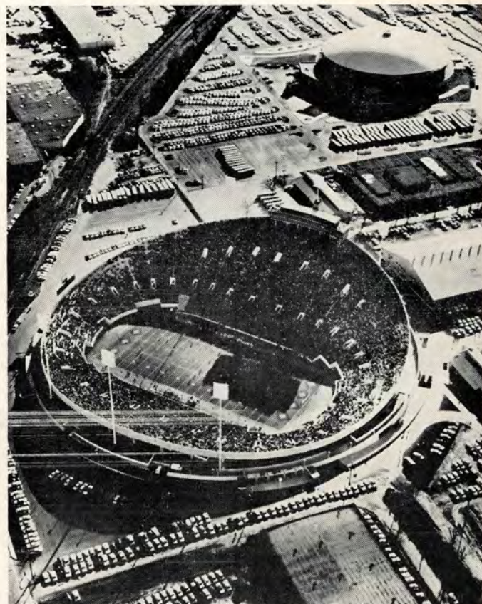
AIR VIEW OF MEMPHIS MEMORIAL STADIUM
