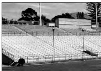
Bleachers on the east side of Alex G. Spanos Stadium were expanded twice in the 1970s.
