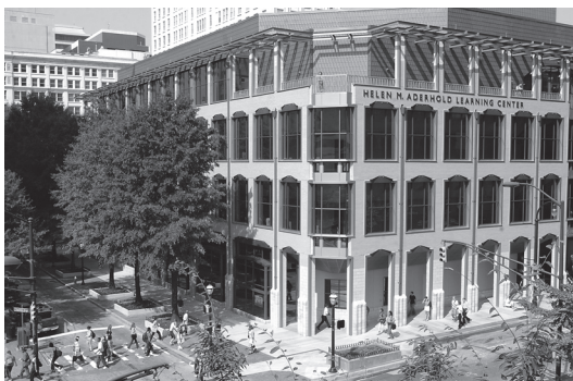
The Helen M. Aderhold Center provides modern classroom facilities in the heart of Georgia State's downtown campus.
