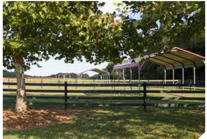
▼ New covered overhangs for horses in pens providing shade and shelter.
