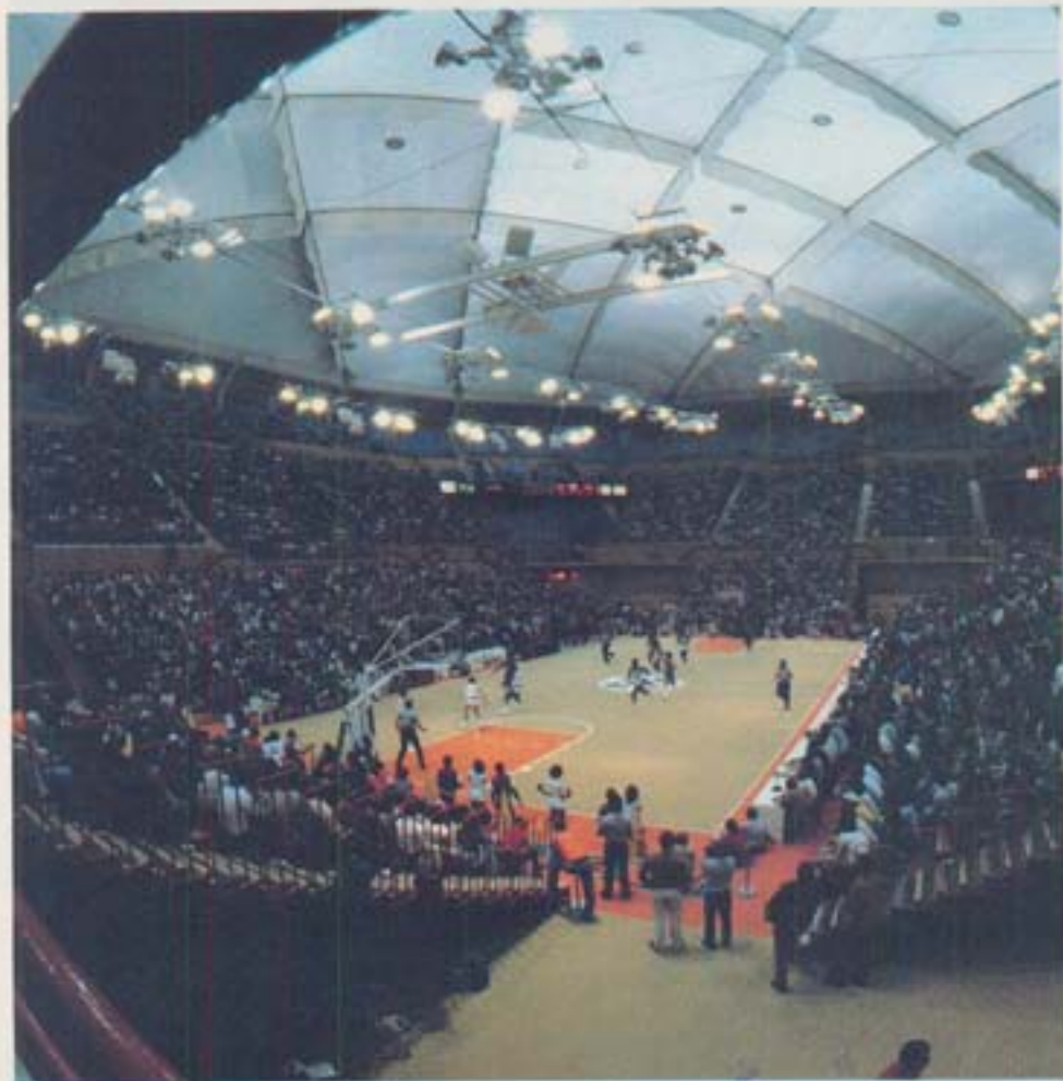
The 12,000-seat main arena of the O'Connell Center (Left) serves as home for the Gator basketball team, as well as a place to hold concerts, banquets and commencement exercises. The Fiberglass roof is suspended by four huge fans that blow heating and cooling air to keep it aloft at all times.
