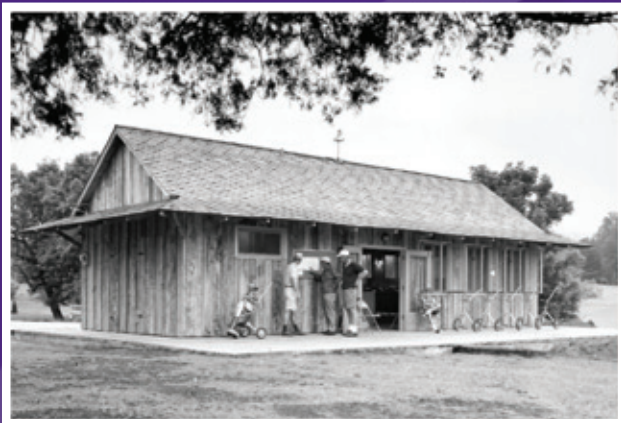
Built in the late 1960's as shown above, the Furman Pro Shop has been expanded twice to include offices and locker rooms.
