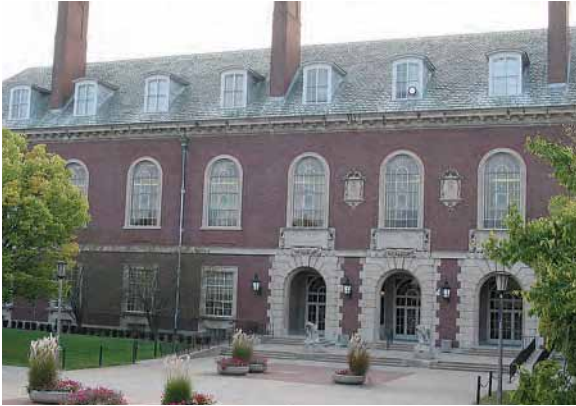
Above: Front view of the Illinois Main Library
