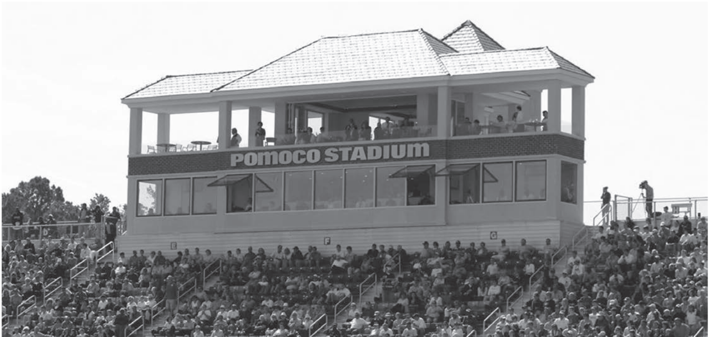
POMOCO Stadium's Perry Press Box
