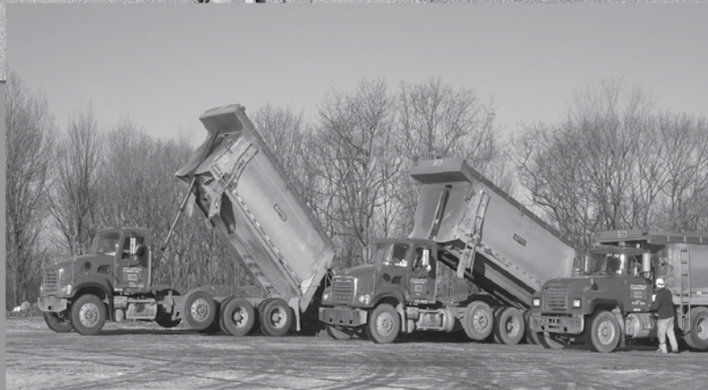
Aggregate materials & delivery
