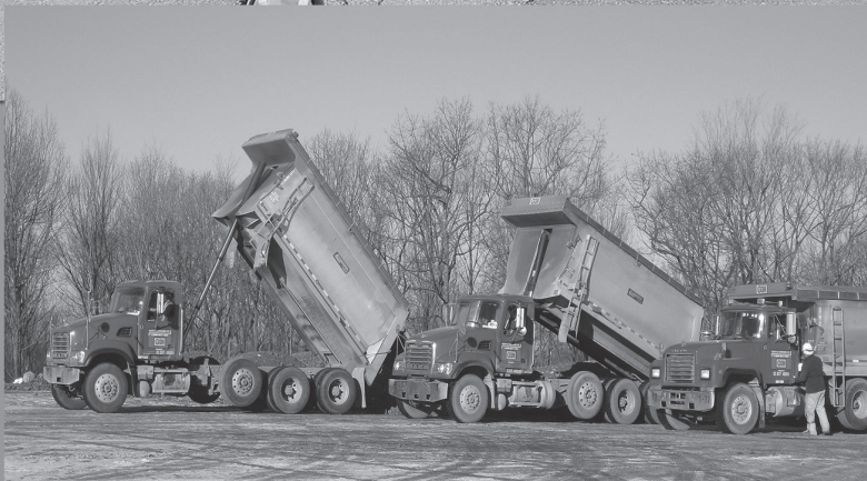
Aggregate materials & delivery
