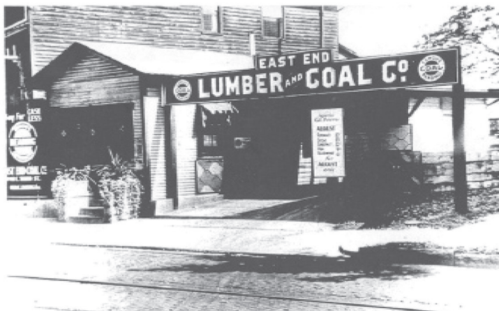
940 E. Third Street (Original Structure)
