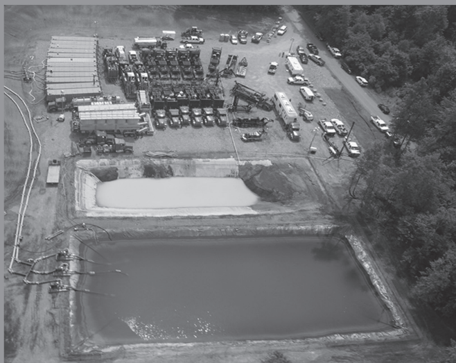
Well pads & impoundments
