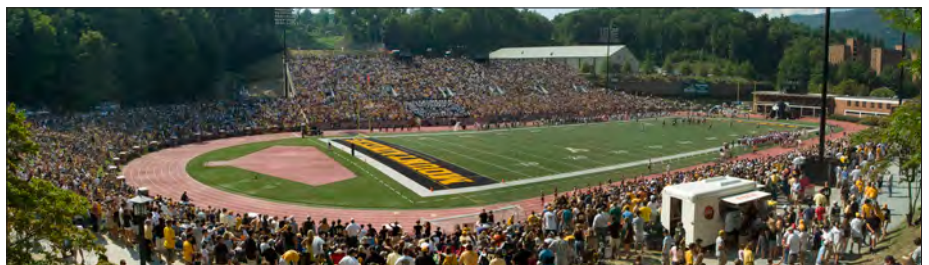
Prior to the 2007 season, the press box was removed from the west side of the stadium to make way for the 120,000-square-foot App State Athletics Center. Following the '07 campaign, construction began on a 4,400-seat upper deck on the stadium's east side.
