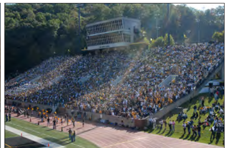
Re-named Kidd Brewer Stadium in 1988, much of the facility remained largely unchanged from 1978 until the beginning of the 21st century. However, additional renovations became necessary when App State began drawing crowds in excess of 20,000 on a regular basis.
