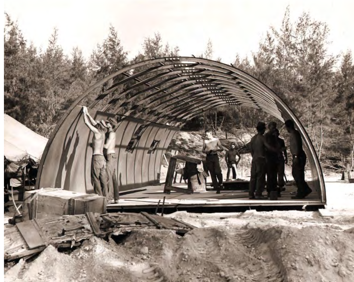
U.S. Navy Seabees assemble a Quonset hut at Chu Lai, Vietnam, 1966.
