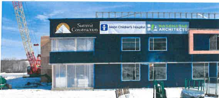
Akron Children's Hospital Health Center Construction
