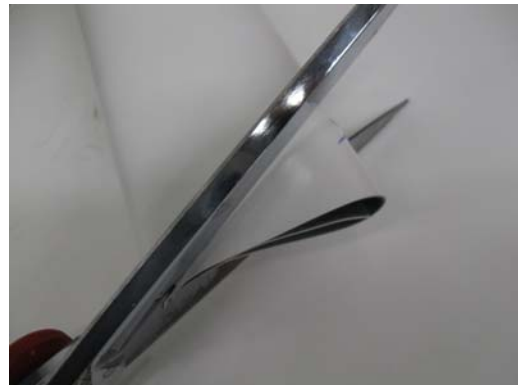
Cut membrane at measured angle.
