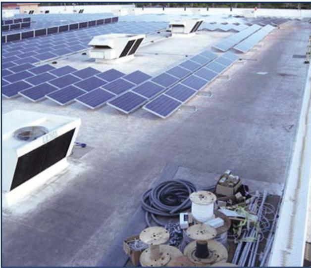
Photo 1 – New TPO roof damaged during PV installation.
