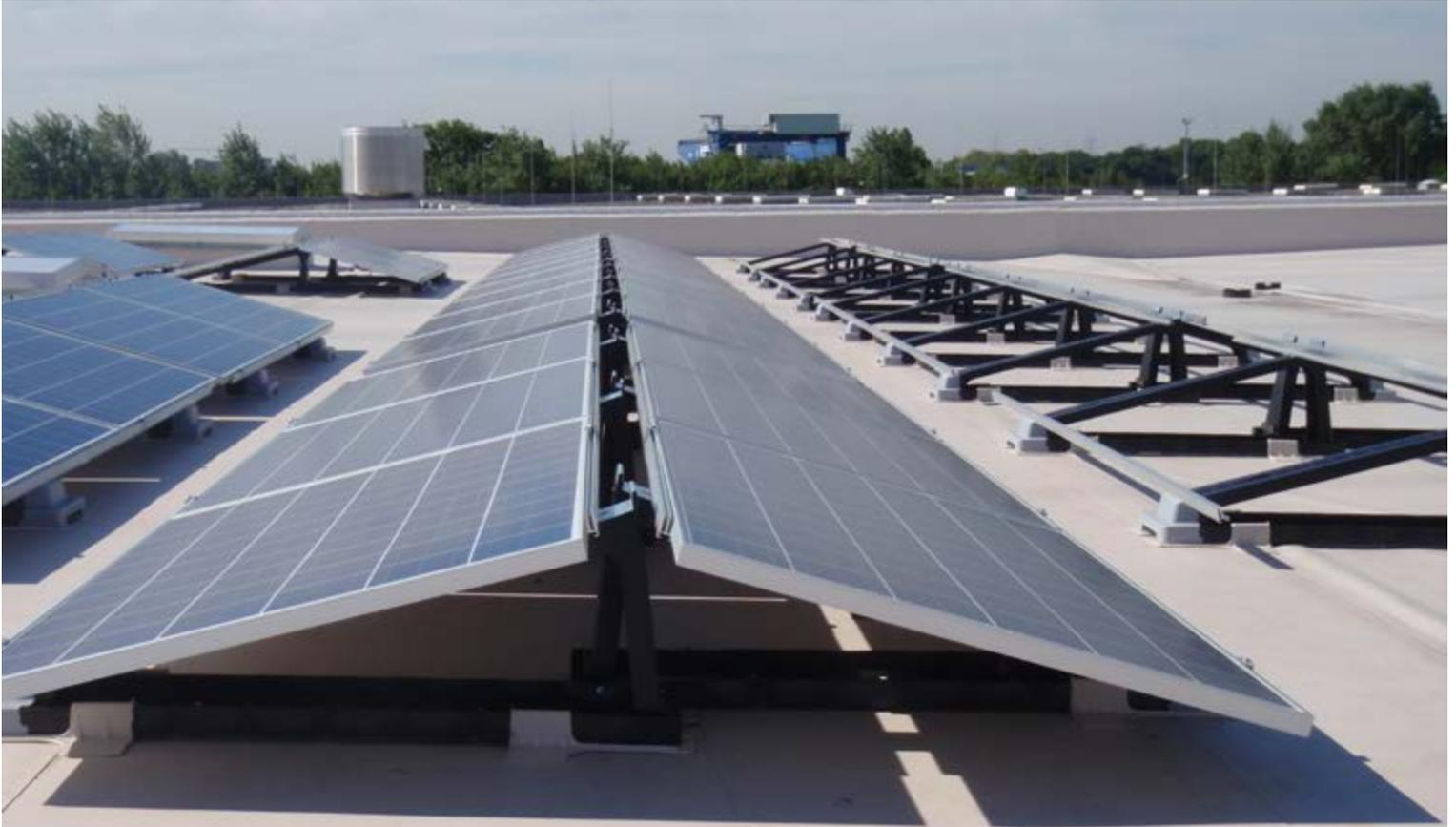
The Sika SolaRoof is a comprehensive, integrated solution incorporating the proven performance of Sarnafil roof assemblies with the Sika SolarMount-1 - an innovative, non-penetrating, engineered solution for long-term securement of solar rooftop photovoltaic.
