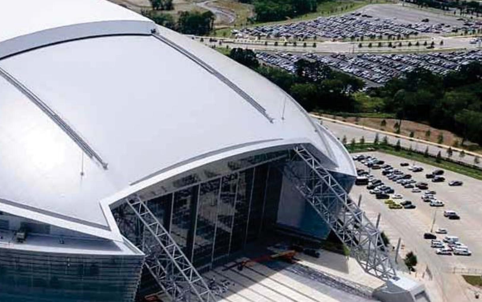
▲ Sika Sarnafil's EnergySmart Roof system, totaling 640,000 square feet, was used to cover the massive fixed dome and several smaller, auxiliary roofs at Cowboys Stadium in Arlington, Texas.
