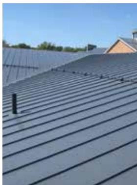
When the Wogaman School decided to replace its shingle roof, the consultants recommended the Sarnafil® Décor Roof System in lead gray on this very visible roof. Harold J. Becker Company, Inc. began the installation of the 850,000 sq. ft. roof in mid-August, 2013, but had to suspend the work in December, due to winter weather. In March the project started again and double crews worked until completion in October. The project required approximately 17,500 man hours.
